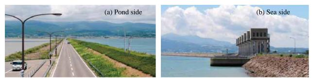
Fig. 2.2 (a) The 7km long Dike separating dam water from seawater, (b) North water gate Photos: ASSEFAW Michael, July 08 2013
