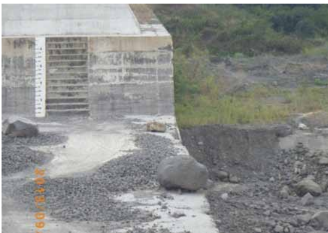
Fig 2.1.3 Upstream of Putih River
