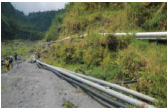
Fig 2.1.10 Complex pipeline water supply system installed in Kuning River
