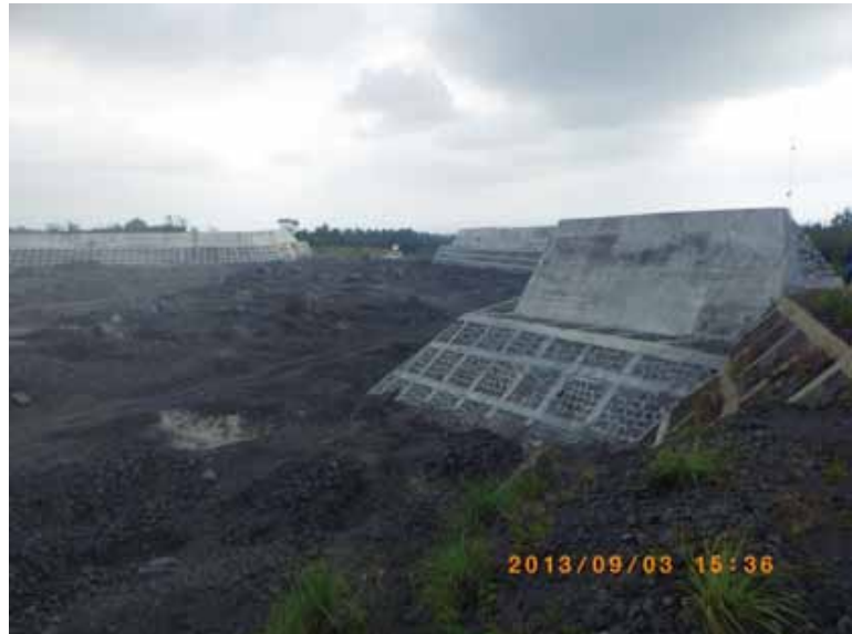
Fig 1.2.1 Sabo dam in upstream of Putih Ruver
